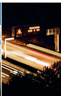
Variable Message Signs and structures
